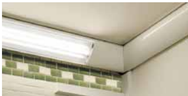
45° corner mounting of the services trunking with double mitre cut.
